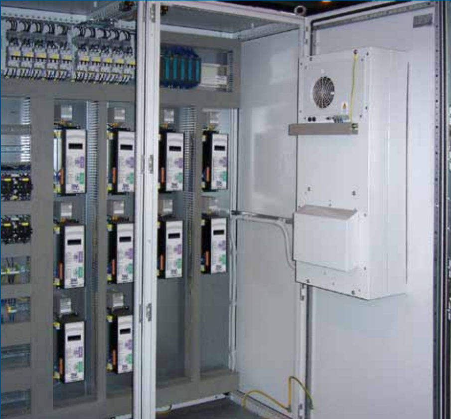
Control panel IP54 with PLC and Air Conditioning
