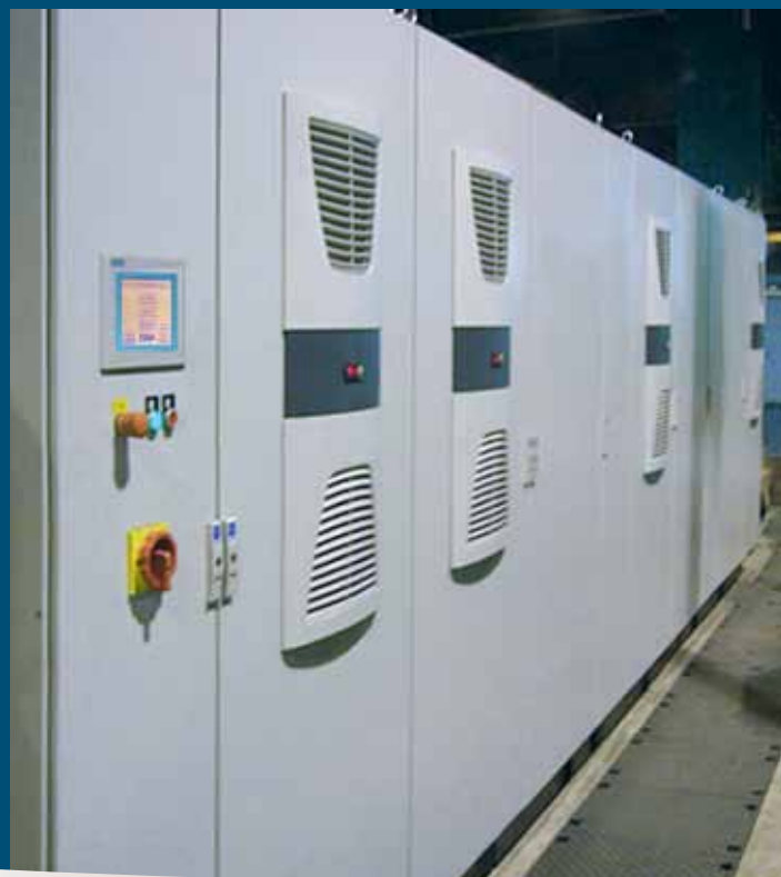
Control cabinet – system – 9 m length with air conditioning and control panel
